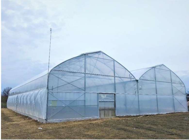
Figure 2. Picture of the installed greenhouse
