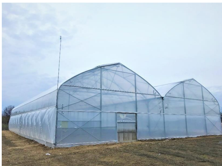
Figure 2. Picture of the installed greenhouse
